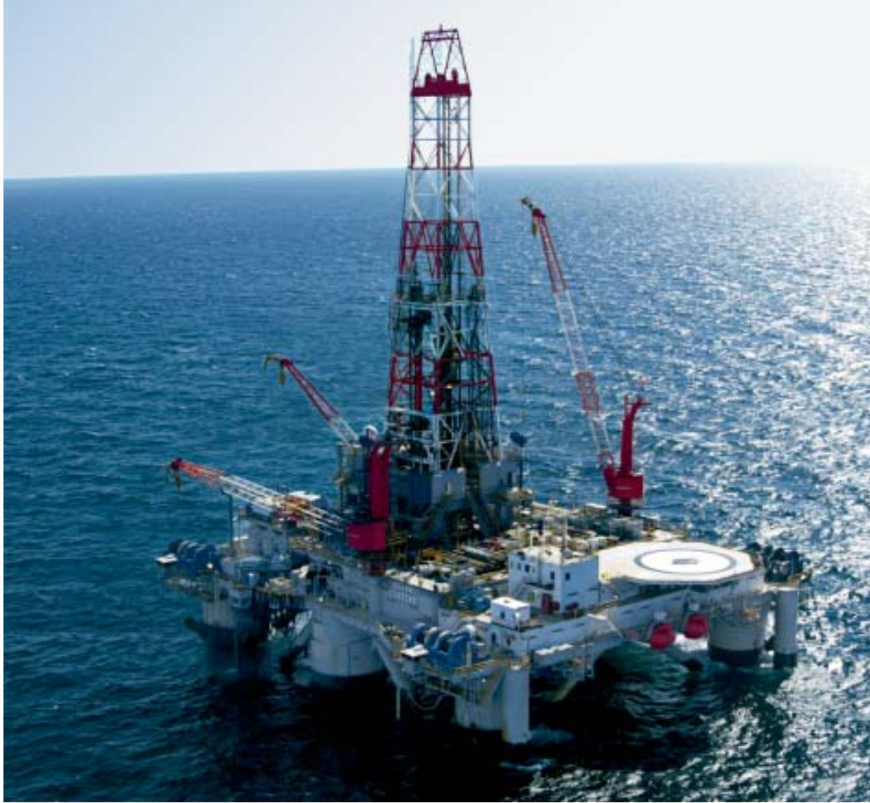
Drilling rig in the Northwestern Field , Gulf of Mexico.
