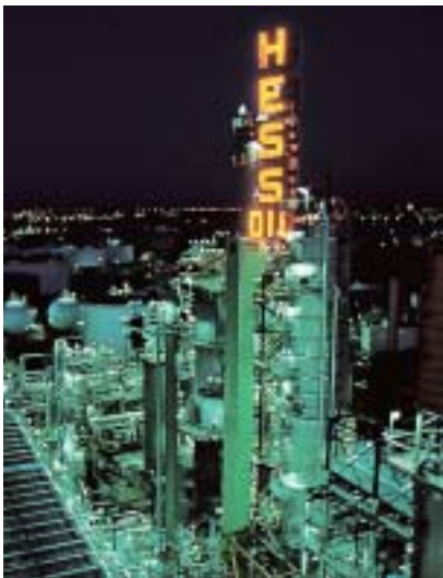
The Port Reading fluid catalytic cracking unit in New Jersey produces high-quality, clean-burning gasoline for northeast markets.
